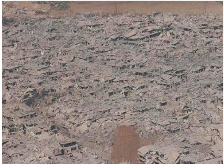
Helicopter view of Nahr al-Bared Camp
